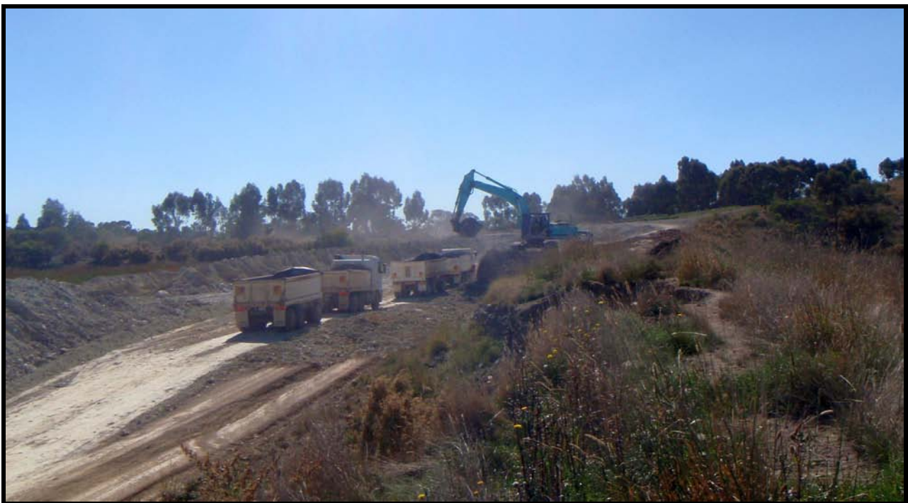
Photo 2 Abigroup Excavating and Trucking from the Eastern Overburden Dump
